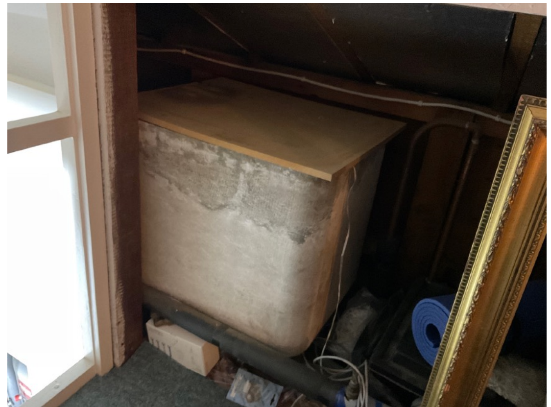
Old header tank: attic and its removal
