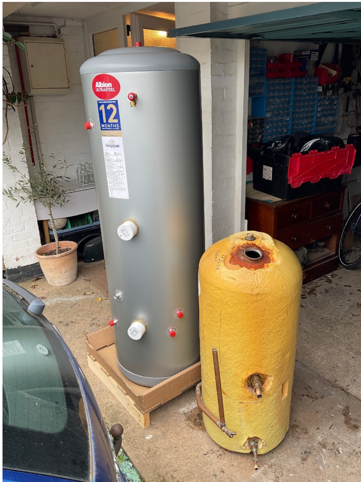
New unvented cylinder beside old vented
